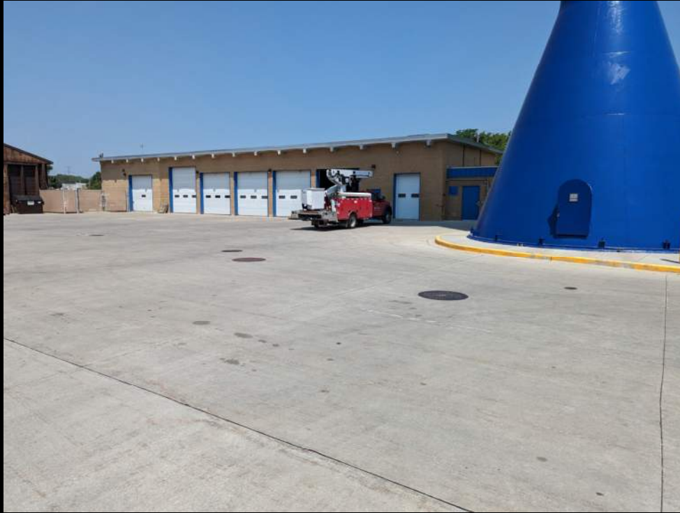
Water Tower Area - NW
