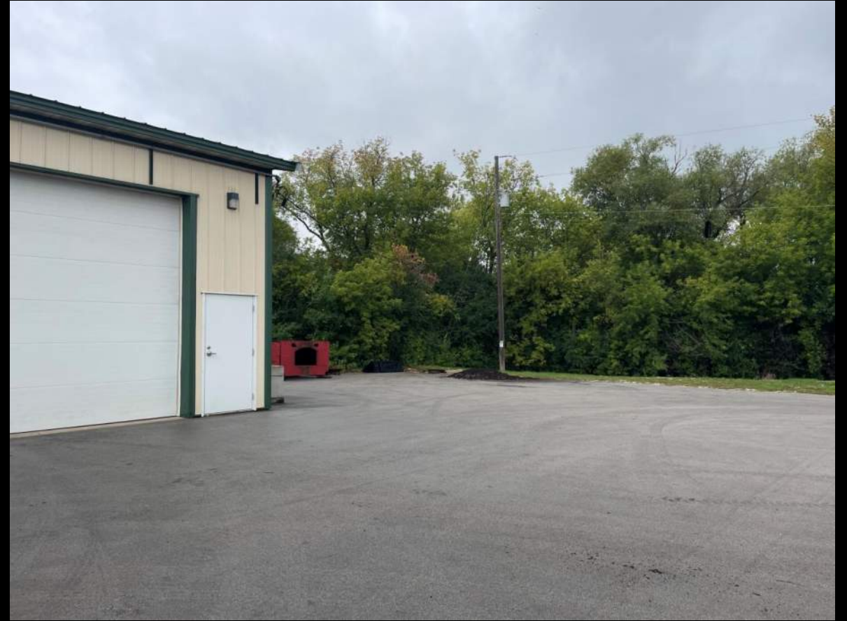
Pavement Area - NW
