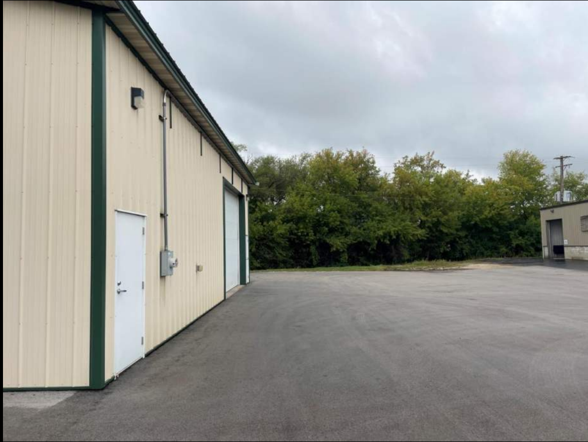
Front of Building - N
