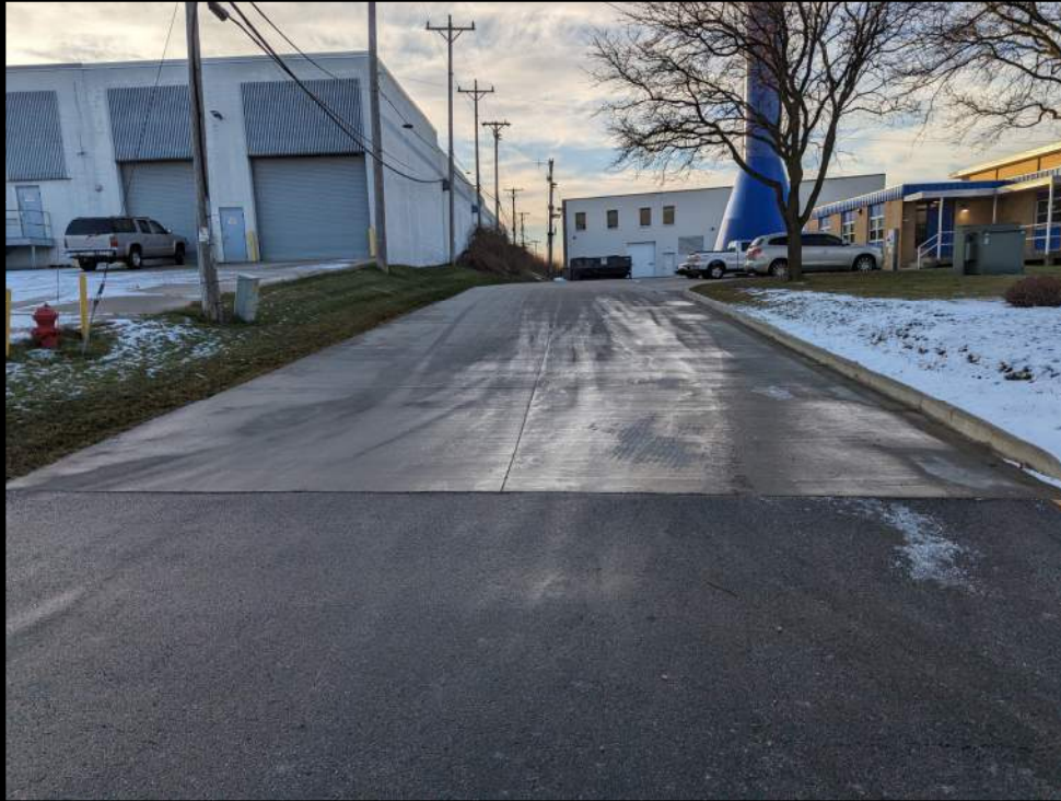
Driveway Area - S
