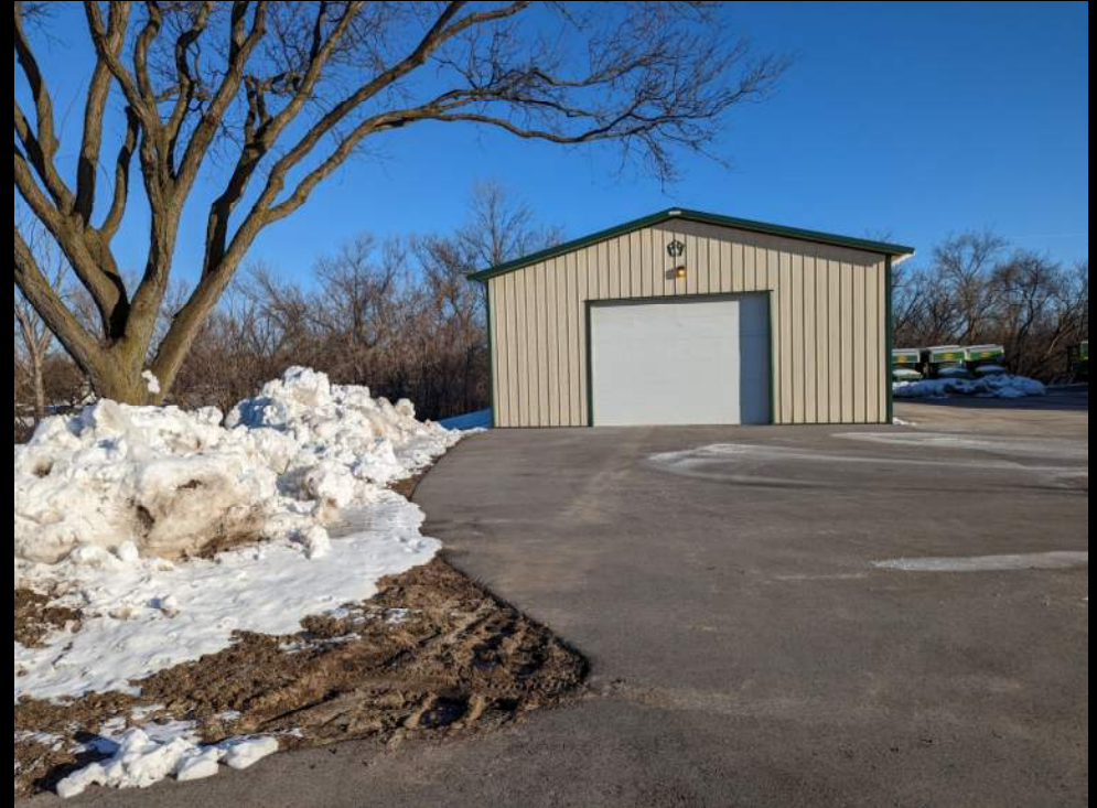
Pavement Area - NE
