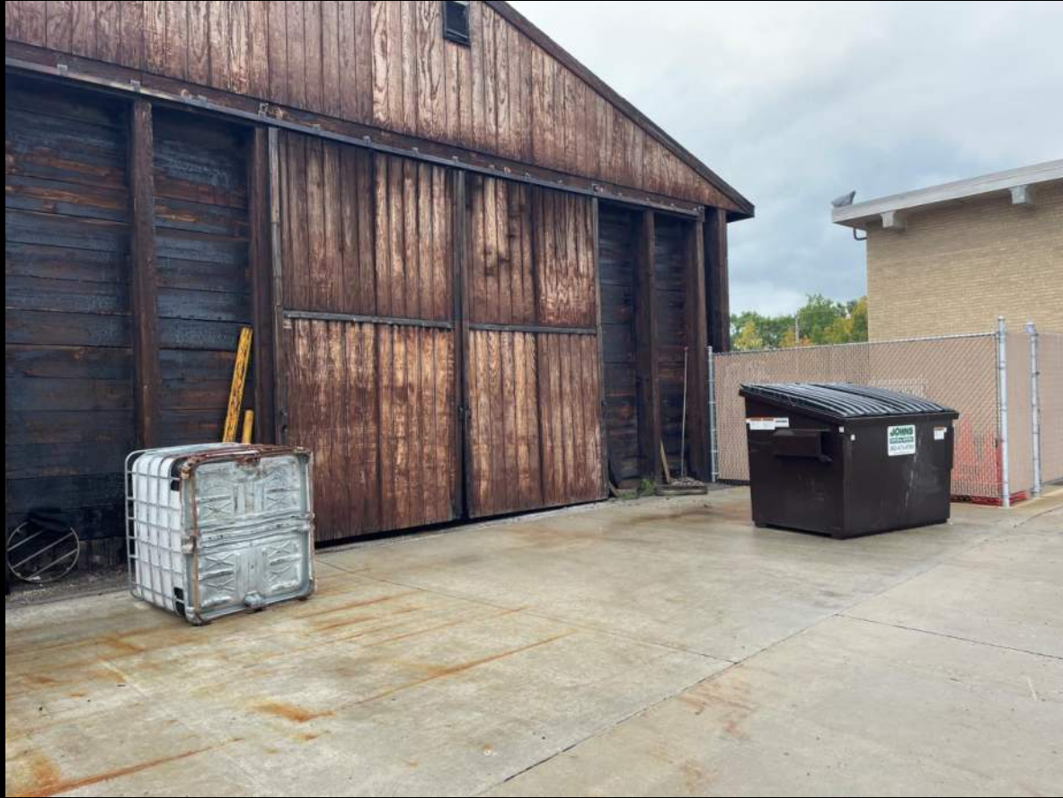
Salt Storage Area - NW
