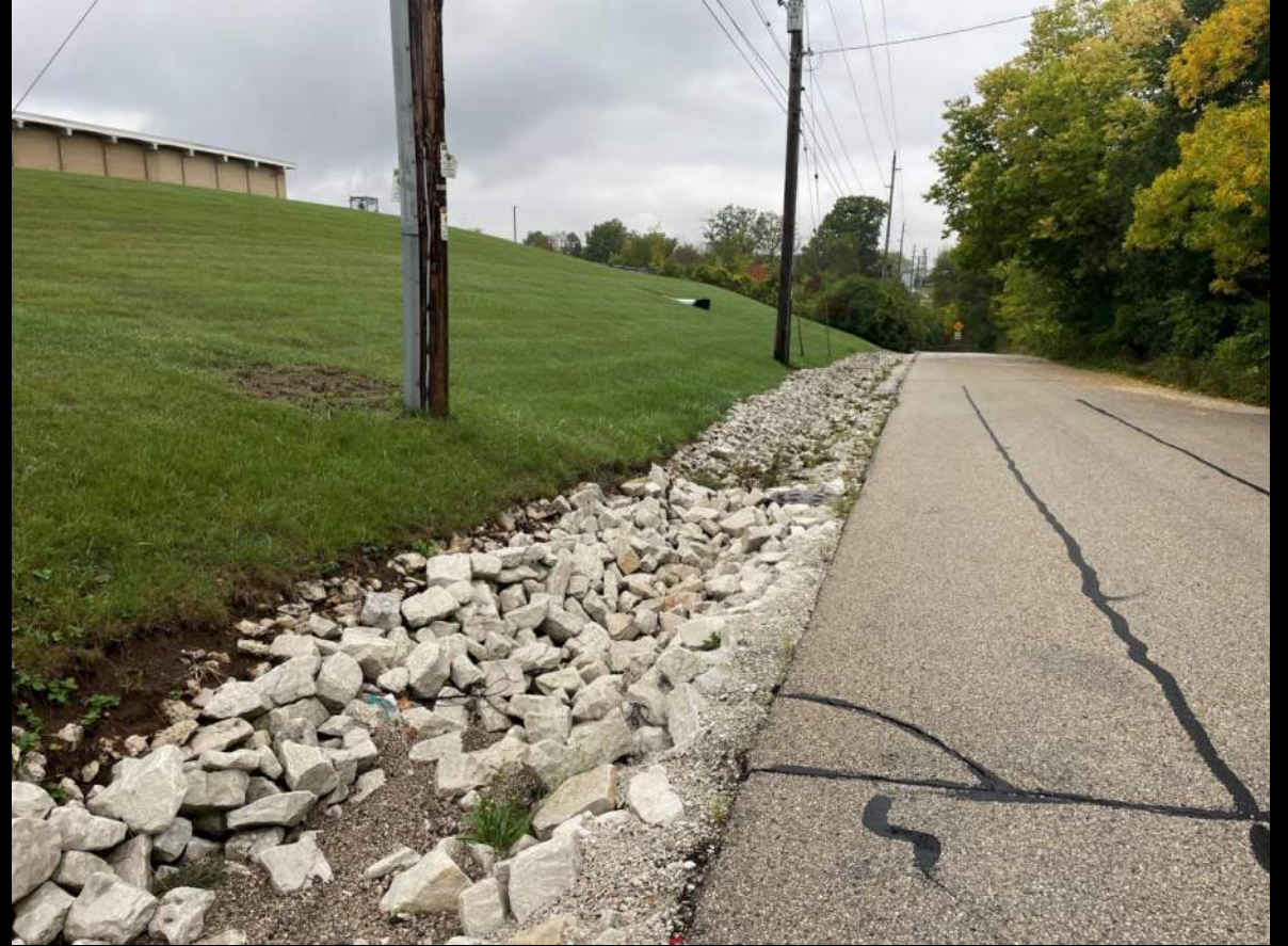
Ditch Area - W
