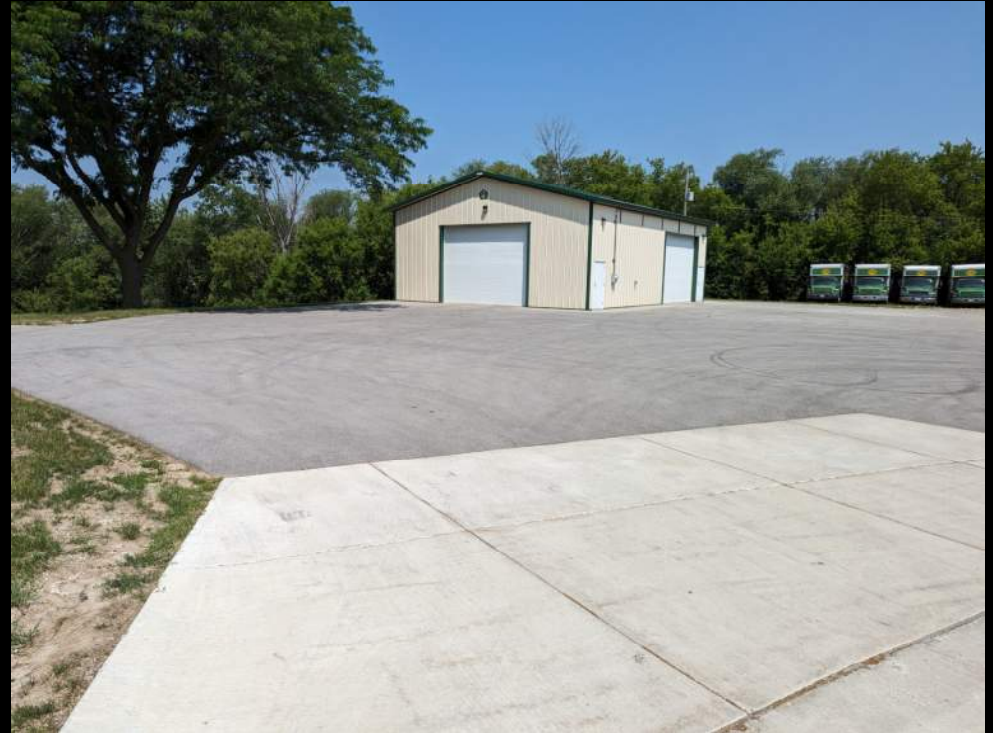
Pavement Area - NW
