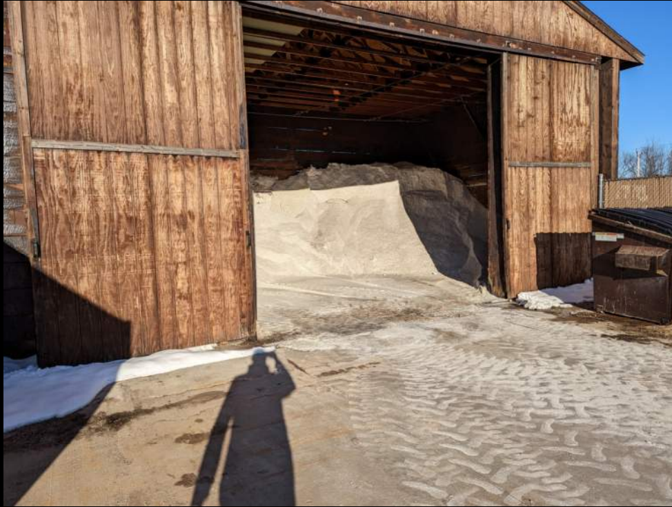
Salt Storage Area - NW
