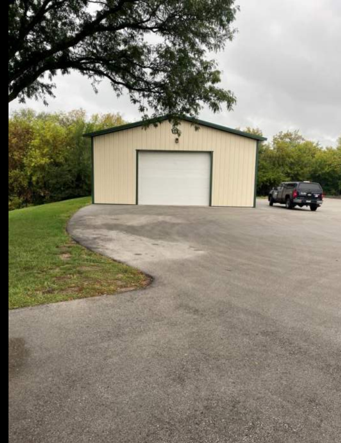
Pavement Area - NE
