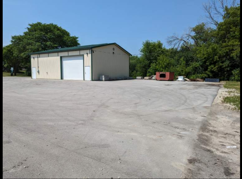
Pavement Area - SW
