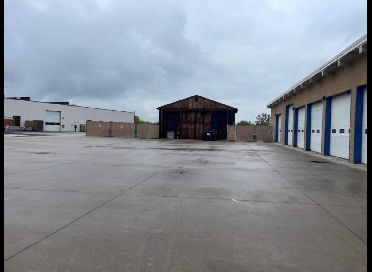
Pavement Area - W
