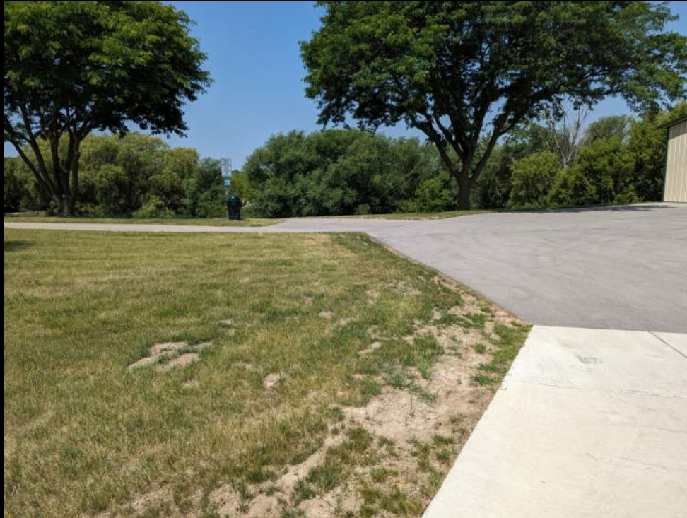
South Edge of Pavement - W
