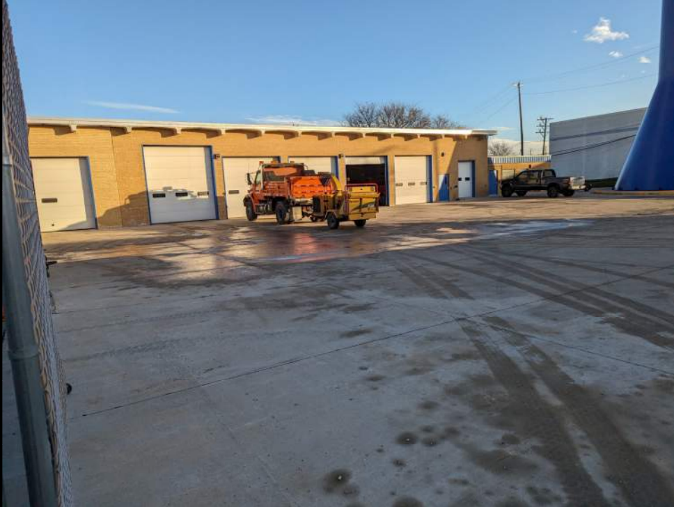
Pavement Area - NE
