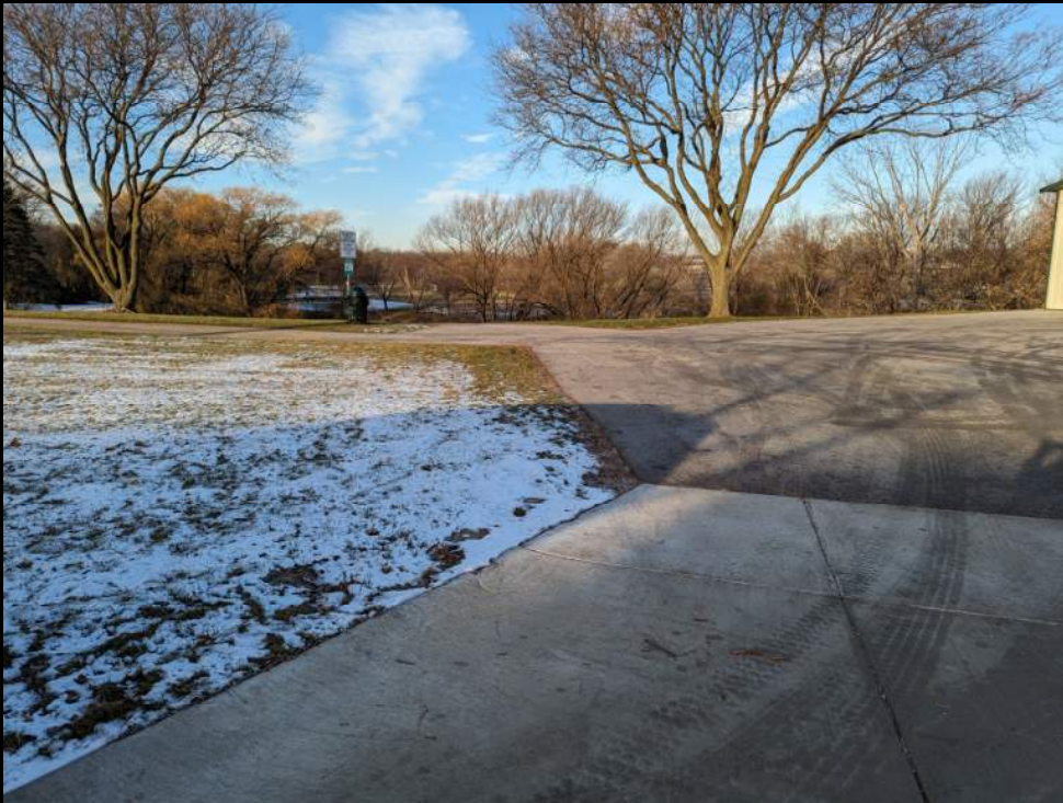
South Edge of Pavement - W
