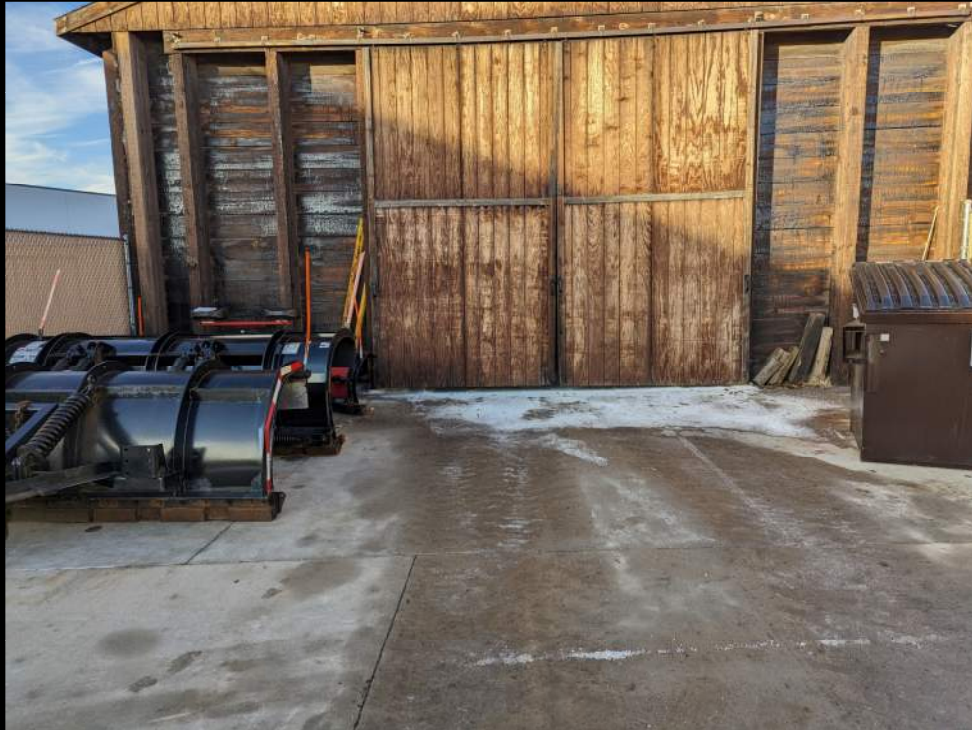
Salt Storage Area - W
