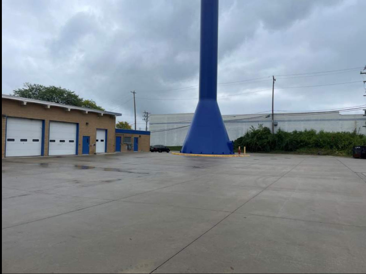
Pavement Area - E
