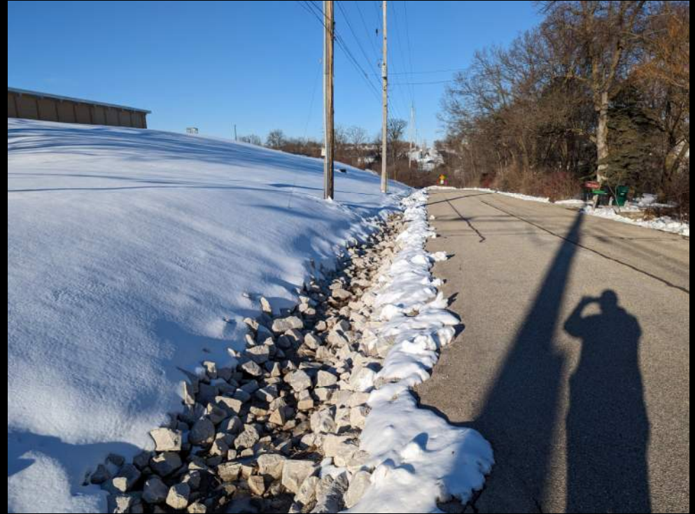
Ditch Area - W
