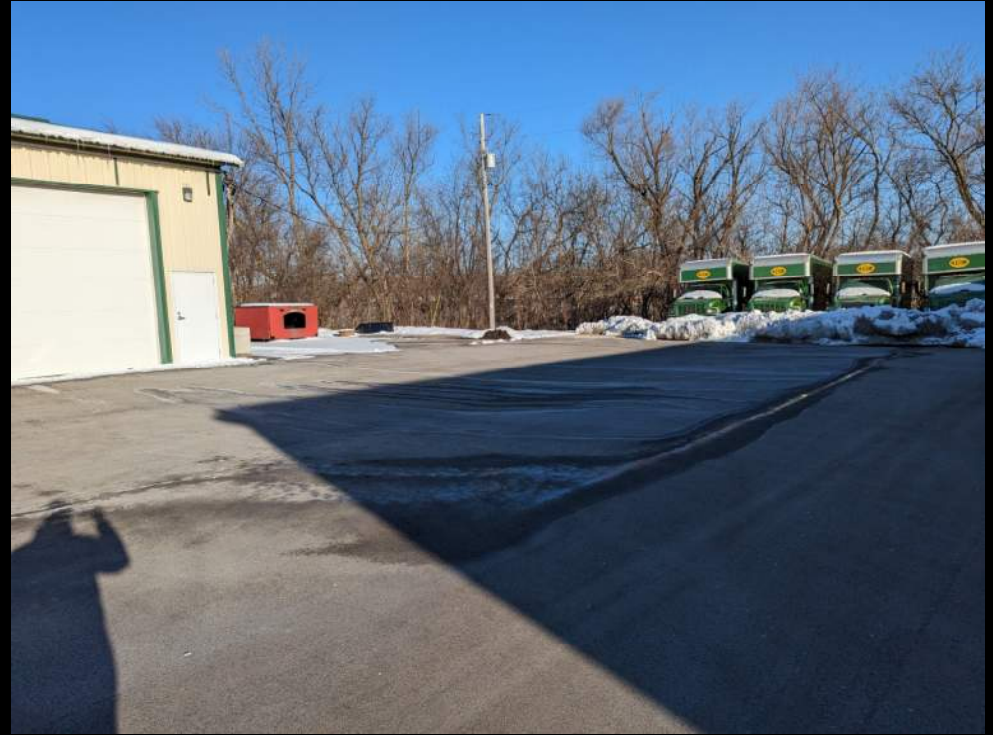
Pavement Area - NW
