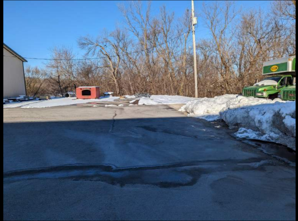
North Edge of Pavement - W
