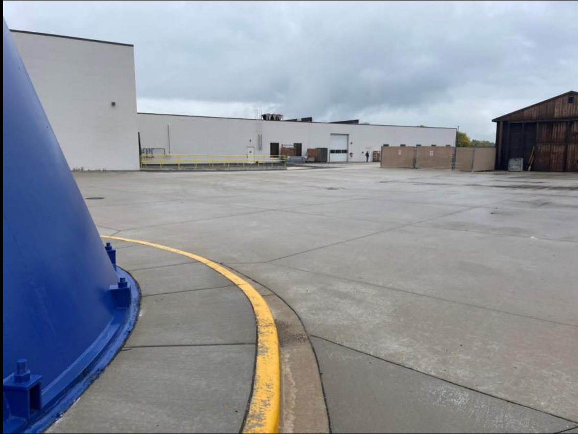
Water Tower Area - W
