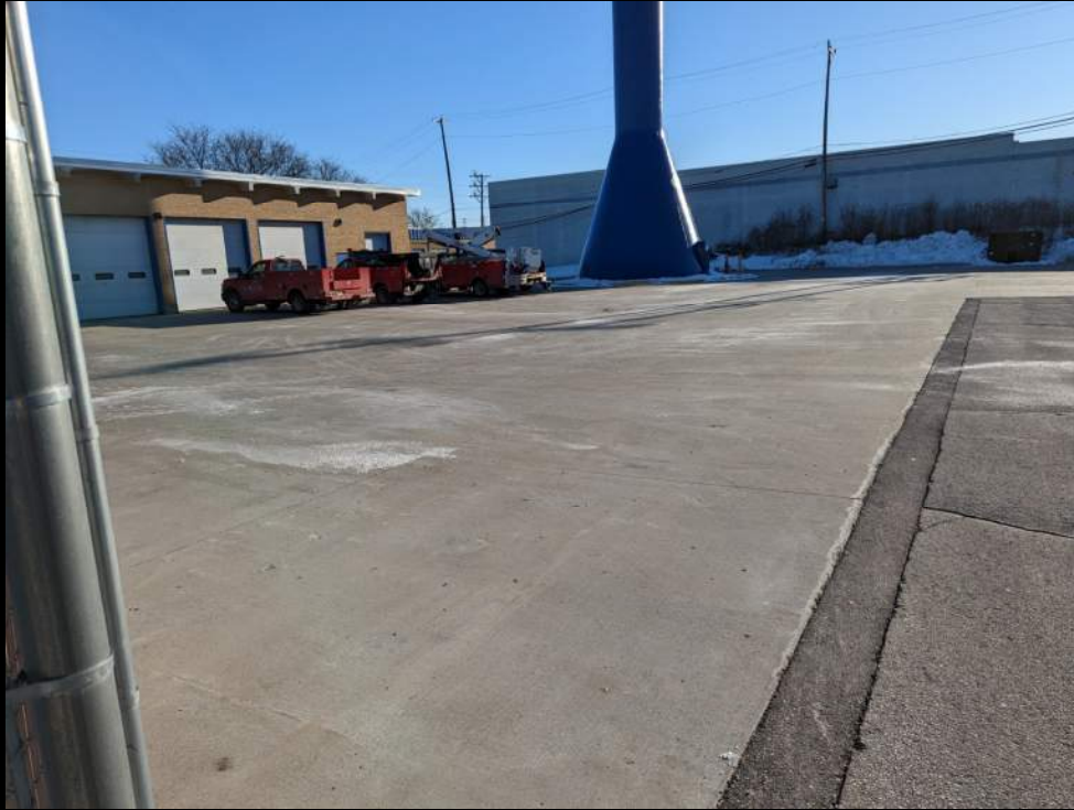
Pavement Area - E
