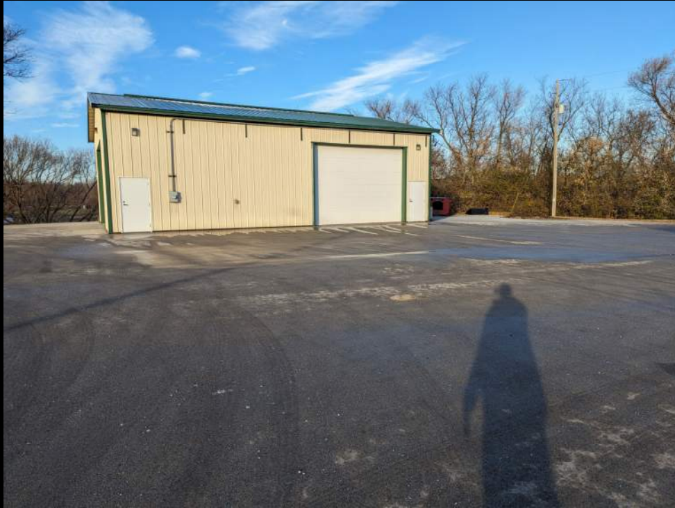
Front of Building - W
