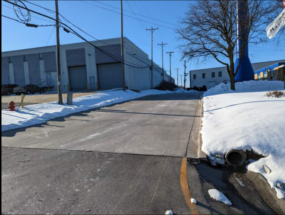
Driveway Area - S
