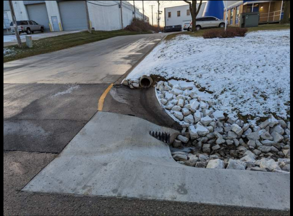
Driveway Culvert - S
