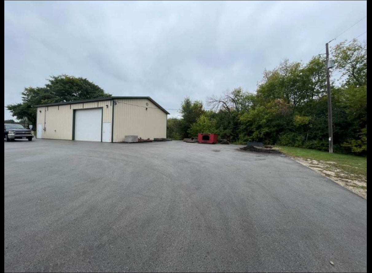
North Edge of Pavement - W
