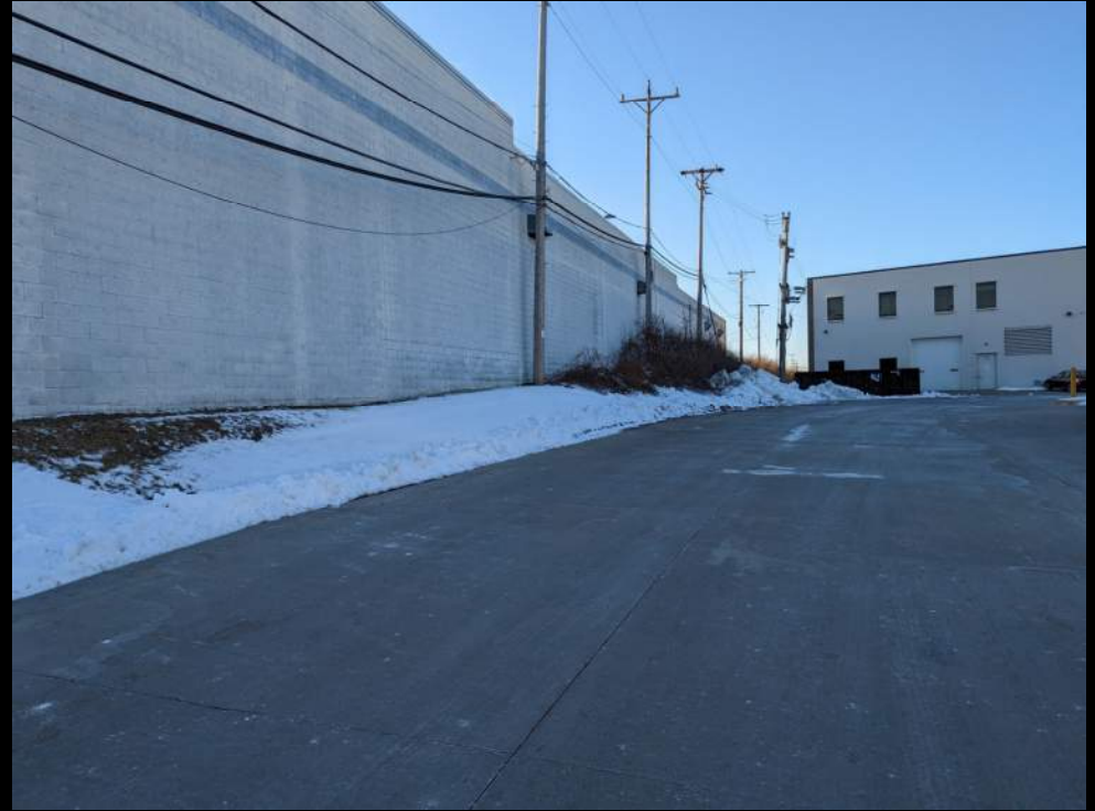
Driveway Area (East Side) - S
