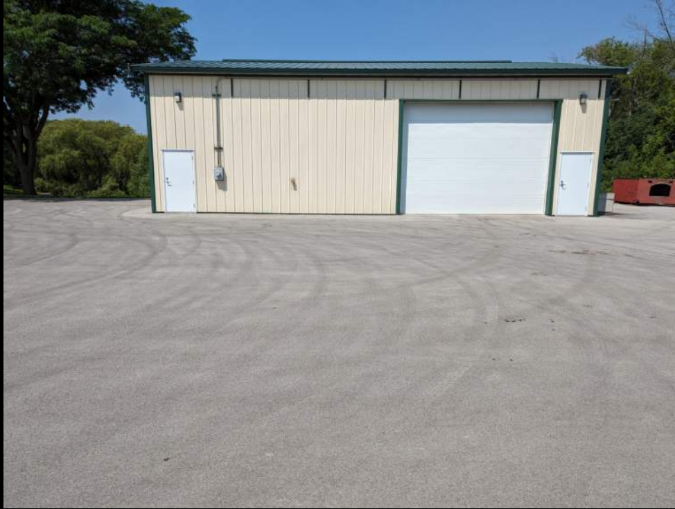
Front of Building - W
