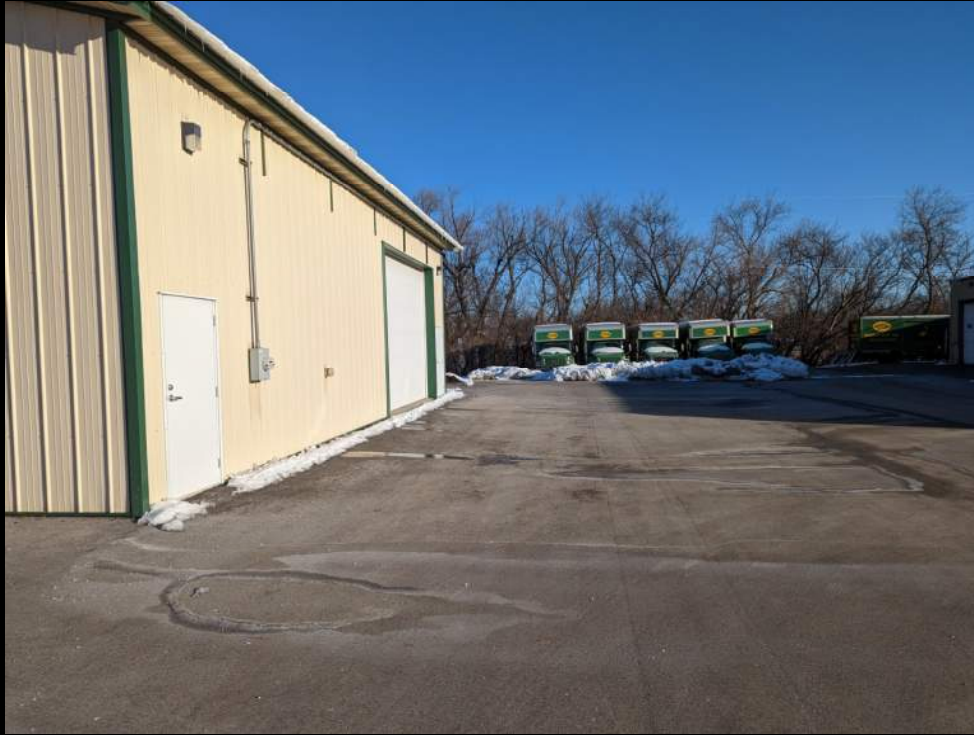
Front of Building - N
