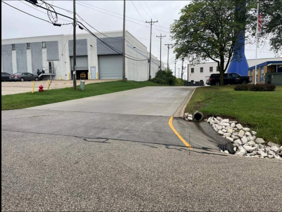
Driveway Area - S
