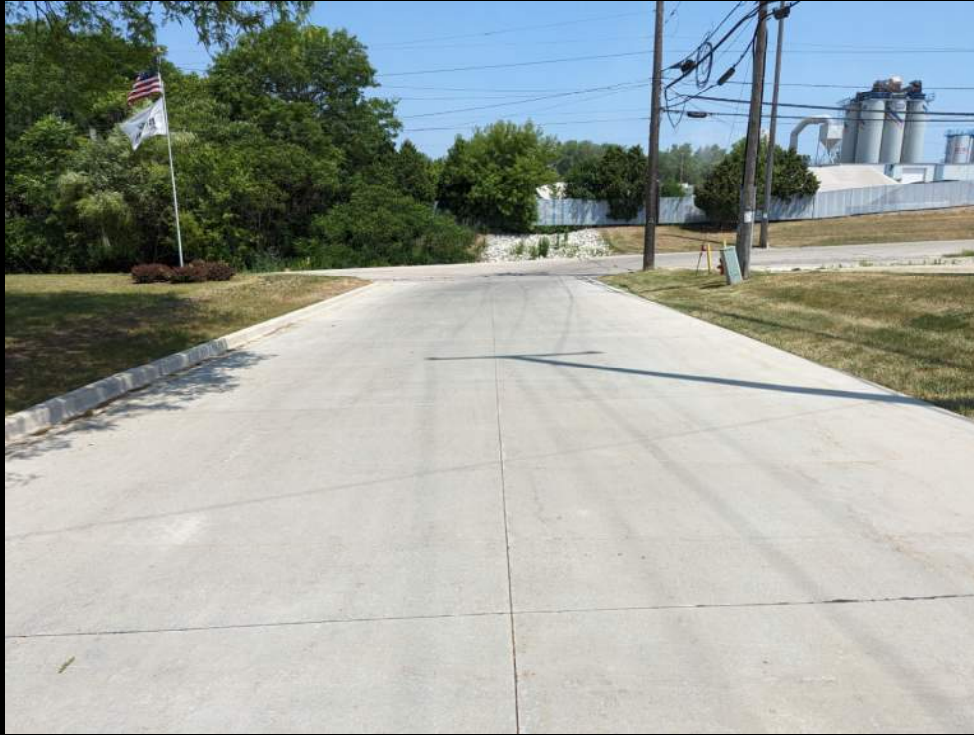
Driveway Area - N
