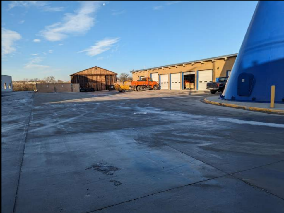
Water Tower Area - W
