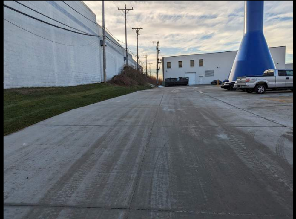
Driveway Area (East Side) - S
