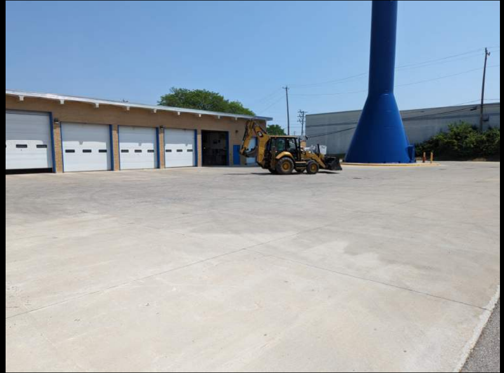
Pavement Area - NE
