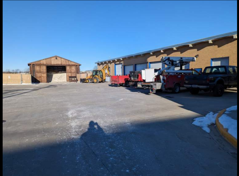
Pavement Area - W
