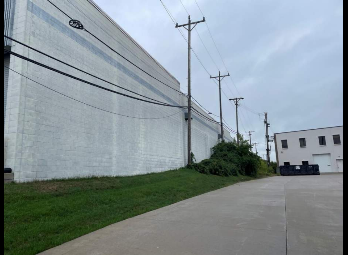
Driveway Area (East Side) - S
