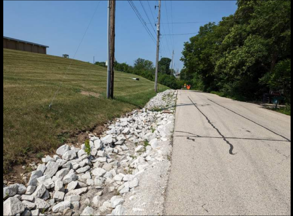
Ditch Area - W
